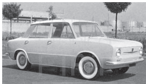
Model “122/540”, design 1a, 1960. An early design suggestion, made in sheet metal, aiming at a shape reminiscent of the 600. The stylistic link between models, proposed for marketing reasons, was actually taken up later on by the 850, the eventual replacement for the 600 in the Fiat range.
