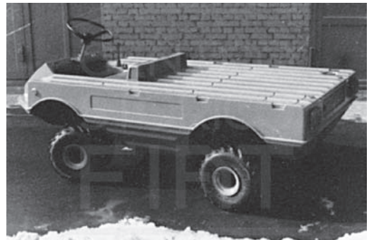
The tipo 17 was conceived as a small transport for use in airports etc. It was derived from the tipo 14 by simplifying the mechanicals. It had a fibreglass-reinforced plastic coachwork. The project was directed by Magnino in the period 1972-74.
